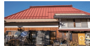
Renovated an old house built in 1929.
